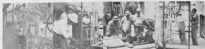
WALTBINE A flow meter is he cuts back on the feed rate of one LOP's electrical coalescers is Operator R. De Kort. CONTEPLANDO UN flow meter mientras el la reduce el feed rate de un di electrical coalescer de LOF is Operator R. Dekort.
